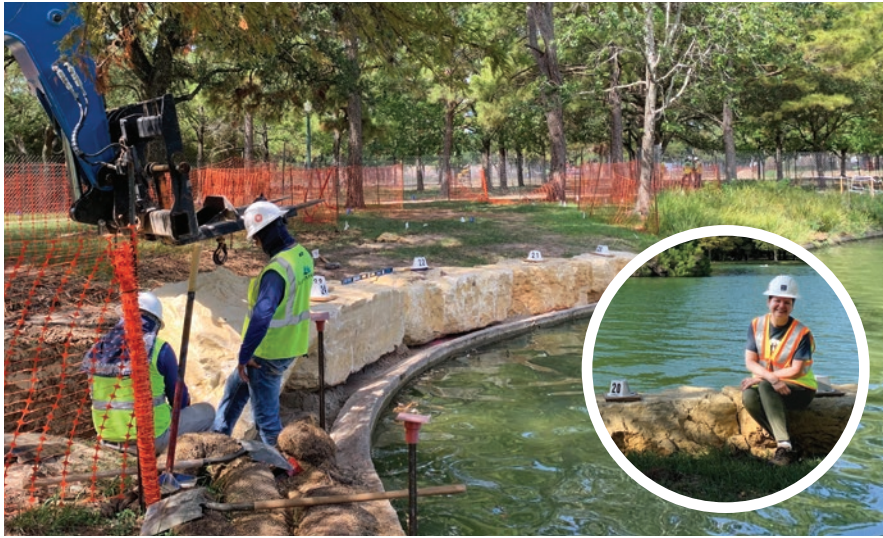
With construction under way, Doreen is already enjoying the new seating!
